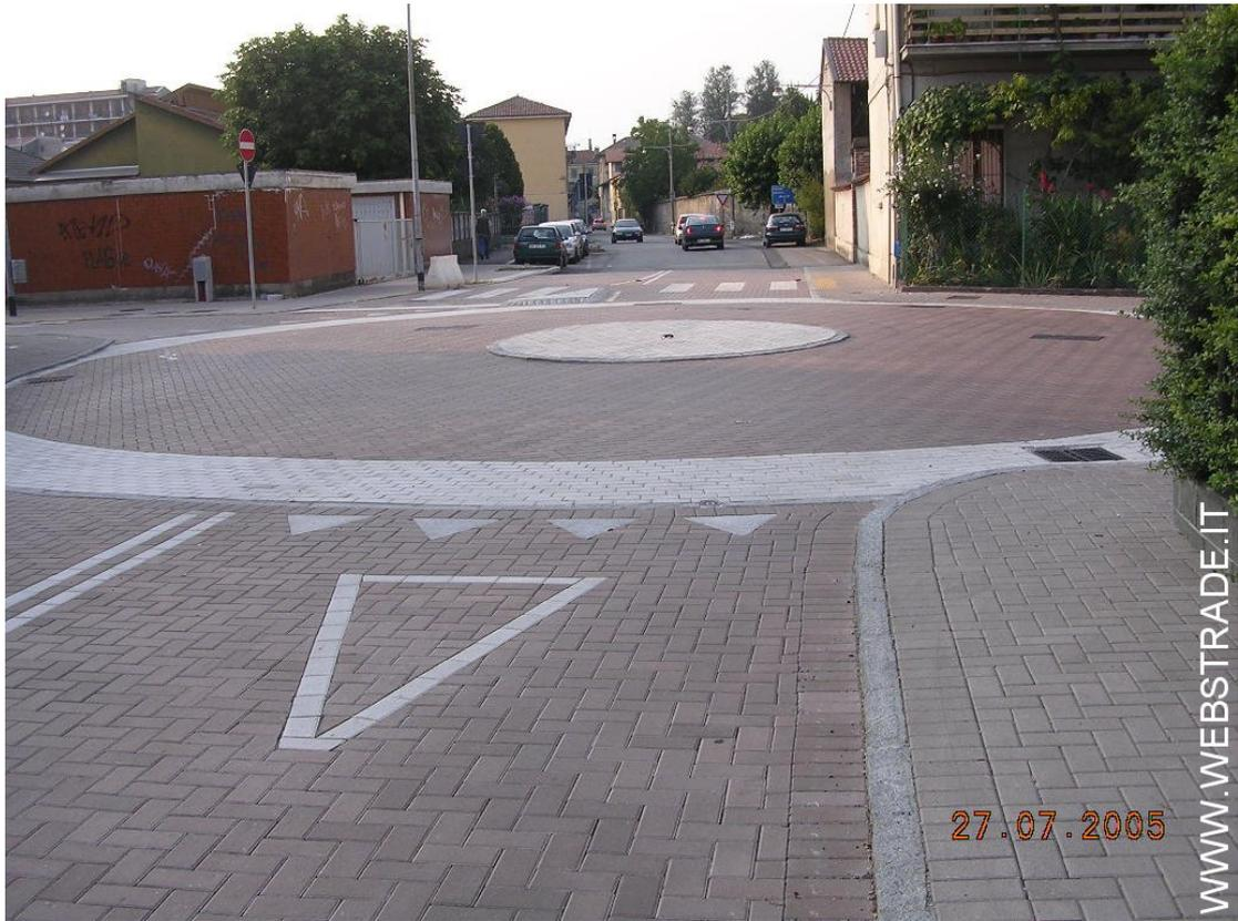
Figure 3- Horizontal road traffic signs using paving slabs
