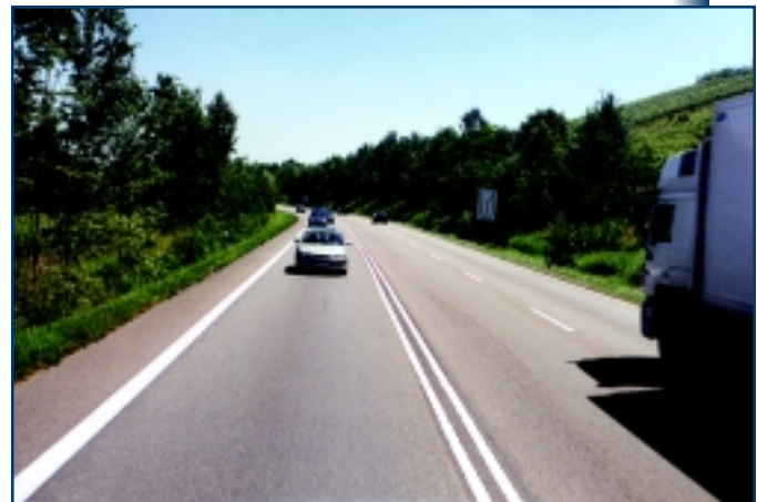
Figure 8. Example of 2+1 road, Germany.
