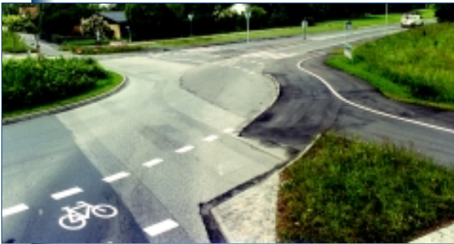
Figure 33. Exclusive bike path on roundabout, Denmark.
