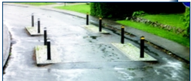
Figure 17. Narrowing with humps, Denmark.
