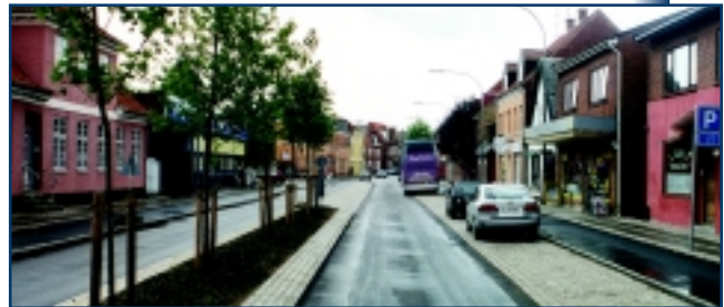
Figure 23. Combination of several traffic calming elements: islands, narrow lanes, and pavement textures, Denmark.
