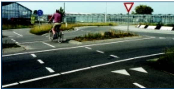
Figure 43. Bike path and roundabout crossing on separate paths, The Netherlands.
