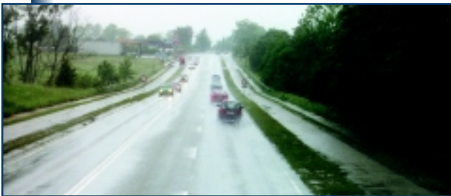
Figure 11. 2+1 road without median separator, Denmark.
