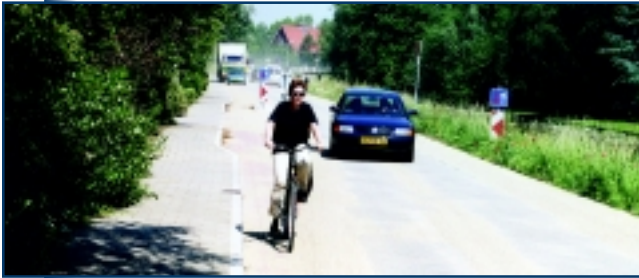
Figure 19. Narrowing by eliminating one lane, The Netherlands.
