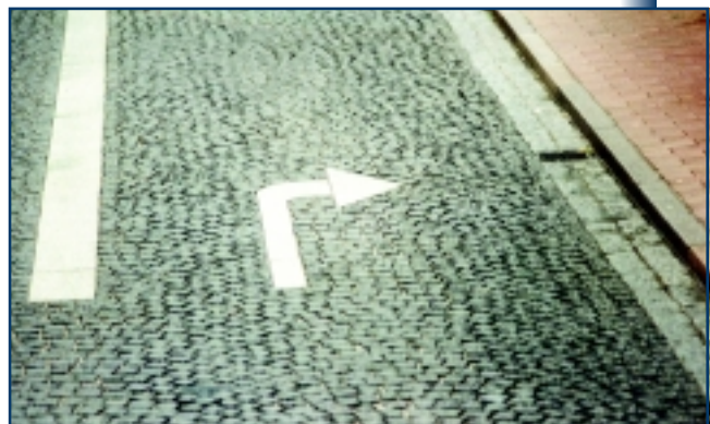
Figure 25. Lane markings as part of pavement texture, Denmark.
