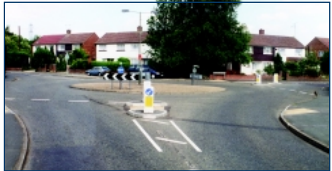
Figure 29. One-lane urban roundabout, England.
